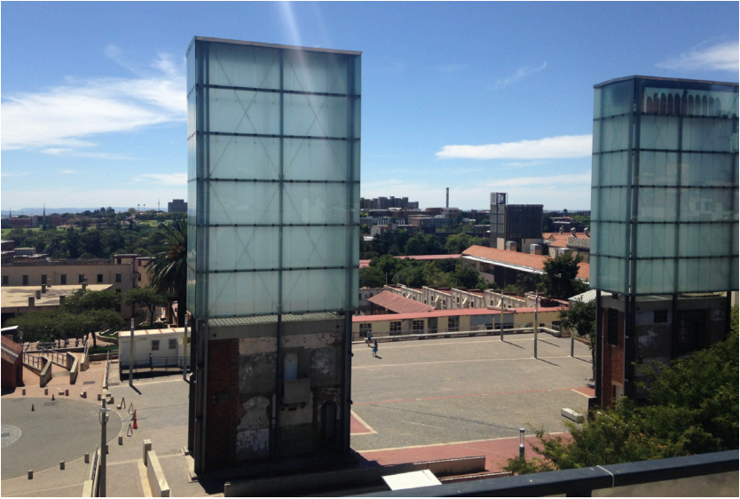
Fig. 3. The original stairwells to the Awaiting Trial Block of the prison complex, since amended with striking lightboxes.
