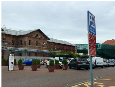
Fig. 2. Osijek Train Station under reconstruction. Photo: Angeliki Sioli, August 2022.
