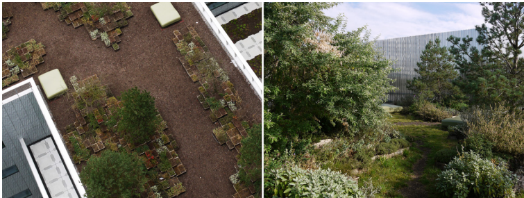
Fig. 5. Toni Areal Roof Garden, Studio Vulkan, Zurich, 2015 (left) A highly unnatural natural place – a pre-cultivated garden in boxes creating an instant garden on call. (right) On opening day of the school the boxes began their process of decomposing. Plants break out, becoming wild and turning the rooftop into an uncontrolled, overgrown setting.
