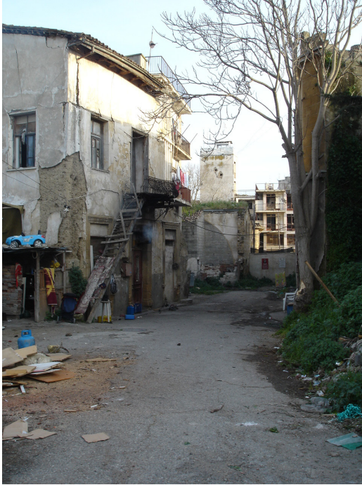
Fig. 11. A dead-end street formed after the divide, photograph by Aslihan Senel, 2013.
