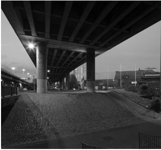
Fig. 4. Underpass built as envisioned in 1965 concept sketches without the footfall and connectivity, Glasgow, 5 December 2017.
