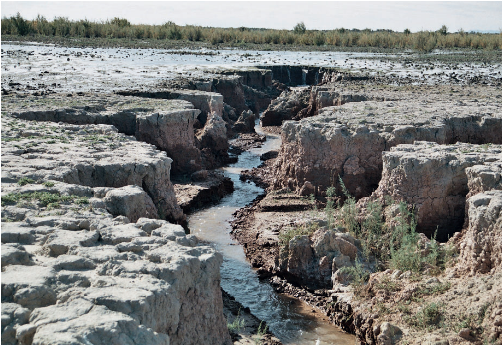
02 Gully formation due to backward erosion. Guanacache 2007 (Photo: H. Paradella)
