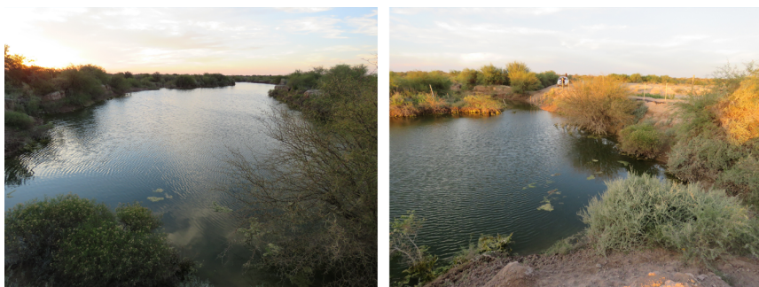
12 La Pasarela project in March 2020 (circled on map). Photo on the left shows the environment upstream of the construction site. Photo on the right shows the construction site
