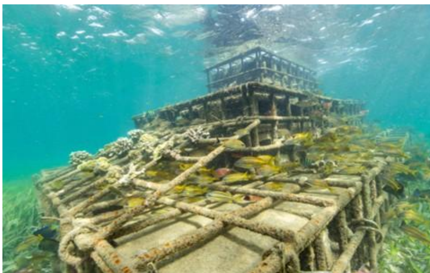
Figure 3. Submerged hybrid breakwater unit in Grenville Bay, Grenada. Source: Tim Calver/Courtesy TNC.
