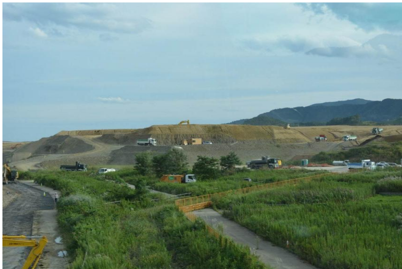
Figure 4: Artificial ground with embankments in Rikuzentakata City.
