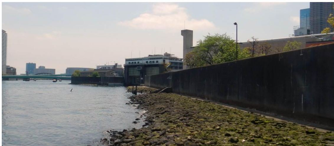
Figure 1: Storm surge embankments in Tokyo Bay
