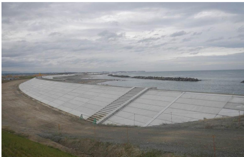
Figure 2: View of a coastal embankment in Iwanuma City. Coastal defence structures are expected to survive after overtopping, reduce the overtopping rate, and delay water intrusion time over land.
