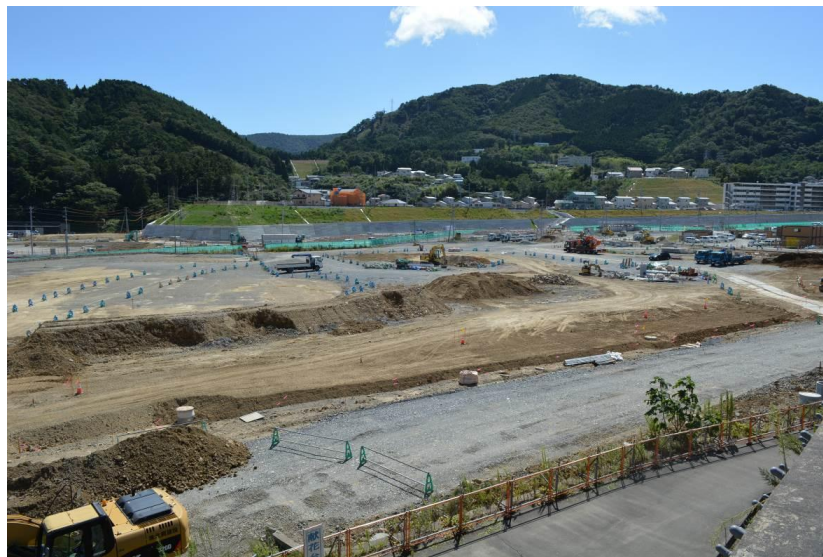
Figure 5: Conversion of old town areas into open space in Onagawa
