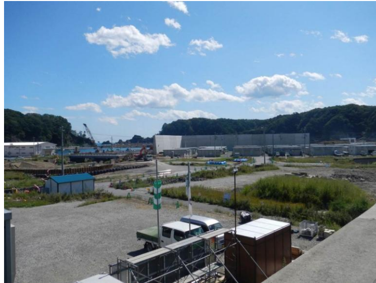
Figure 3: Construction of a new seawall in the Taro area.
