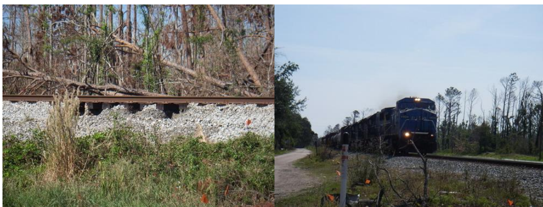
Figure 4. Waveland, Mississippi. Left (Oct 2005): Railroad berm scoured away by the surge. Right (May 2006): Railroad berm repaired and freight trains back in service.
