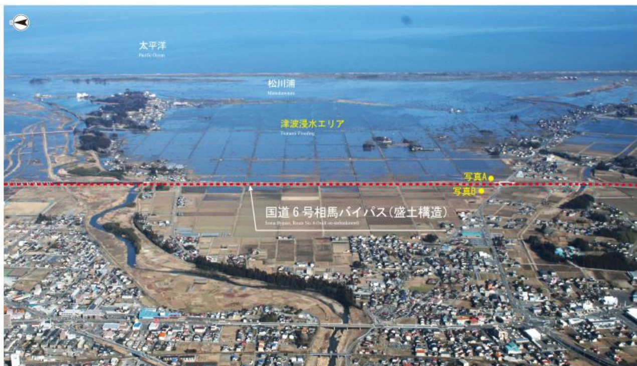
Figure 9. Photo from MLITT (2025) showing the 2011 tsunami primarily confined seaward of the national road #6 Soma Bypass highway embankment in Fukushima Prefecture.
