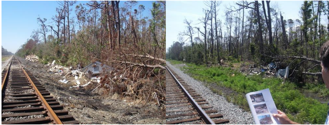
Figure 5. Waveland, Mississippi. Left (Oct 2005): Railroad berm scoured seaward by the surge, and buoyant debris deposited on its seaward side. Right (May 2006): Railroad repaired, and large debris removed. Seaward is to the right.
