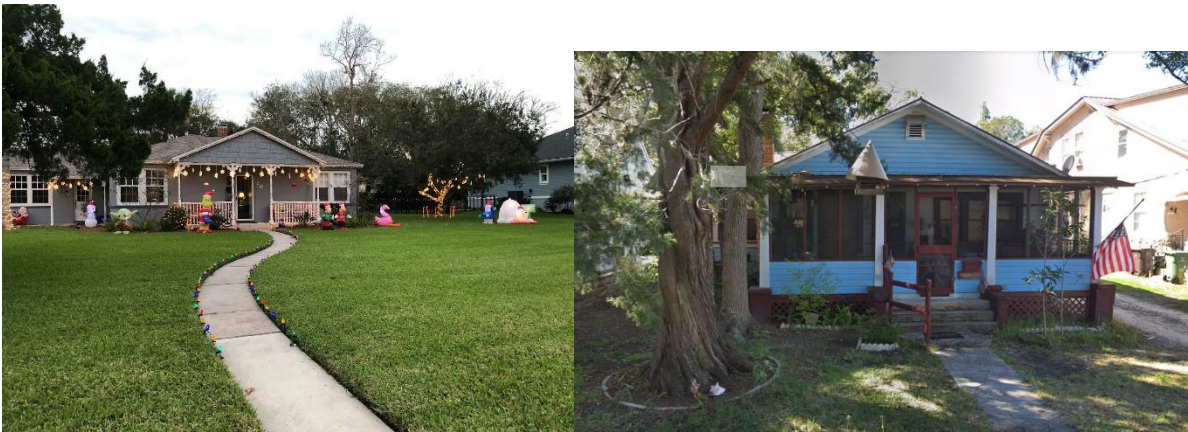
Figure 5. Left. House typical of Davis Shores area. The porch covers a relatively small area in the front, the house is set back roughly 15 meters from the road, and the foundation sits directly on the ground. Right. House typical of Lincolnville neighborhood. The porch stretches the length of the front with room for sitting, the house is set back 5 meters from the street, and the foundation of the house is raised on stilts. Photo from Google Street View with permission of owner.
