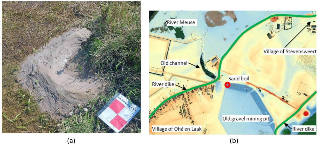
Figure 6: (a) Remnants of a sand boil near St. Annakapel observed after the floods. The sand deposited is relatively fine. (b) ground level in the area of the sand boil (based on the nationwide elevation model AHN3), the dikes are indicated by means of a green line.
