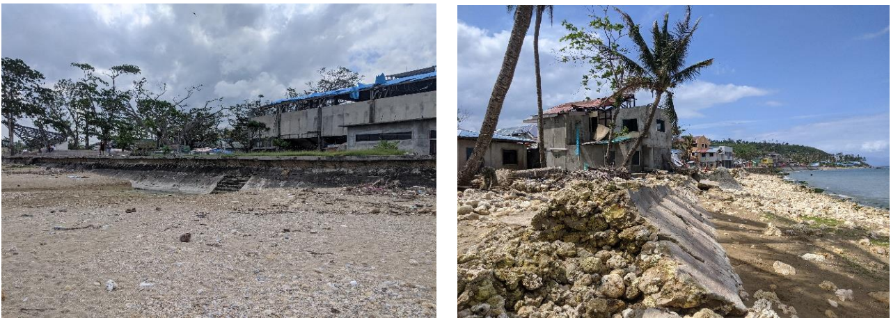
Figure 9. Left. The storm surge reached the top of the seawall in front of Dumanjug market. Right. The storm surge overtopped some of the older seawalls, with scour taking place behind them due to the waves.
