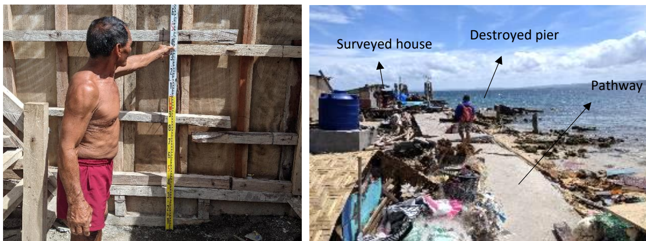
Figure 11. Left. A resident indicates the level of the water in front of the barangay hall. Right. At the right side of the photo is one of the houses surveyed in front of what is left of the pier (structure on the right side)
