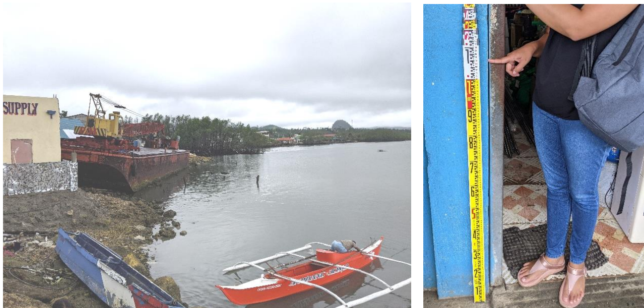
Figure 10. Left. Barge slammed into houses close to Tubigon port. Right. Inundation level in the shop seen on the left side of the figure.
