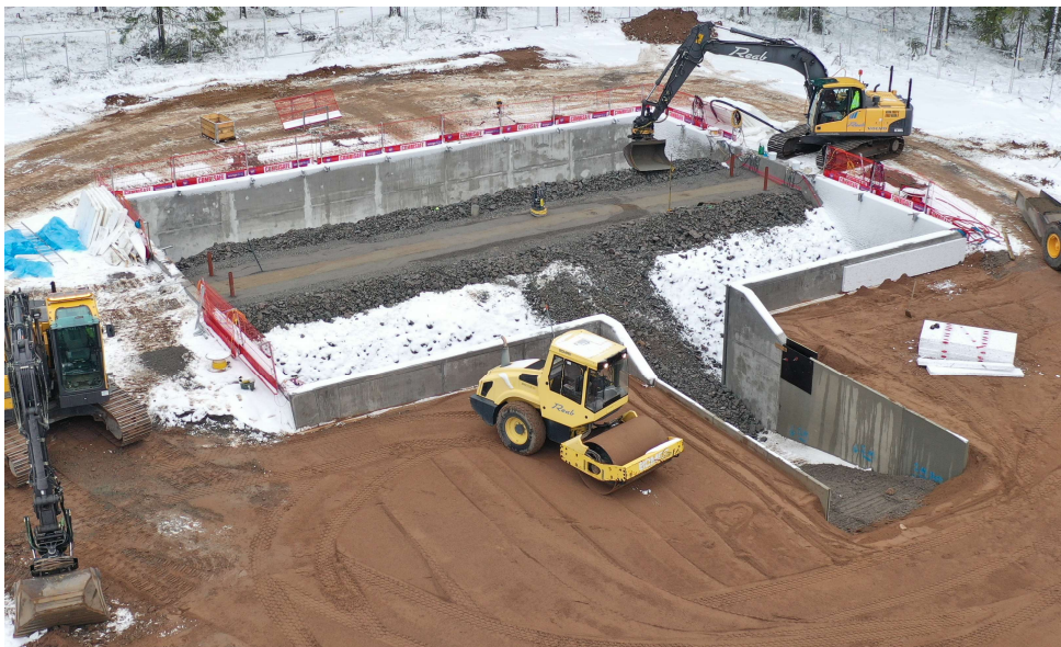
Figure 1. Construction of the test dam inside the concrete containment box in 2019.
