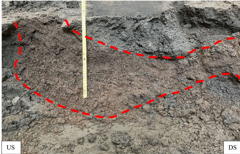
Figure 10. Eroded core soil found close to the wooden cube (between red, dashed lines). The material was coarser on the downstream side than on the upstream side, (Lagerlund and Riaz, 2026).
