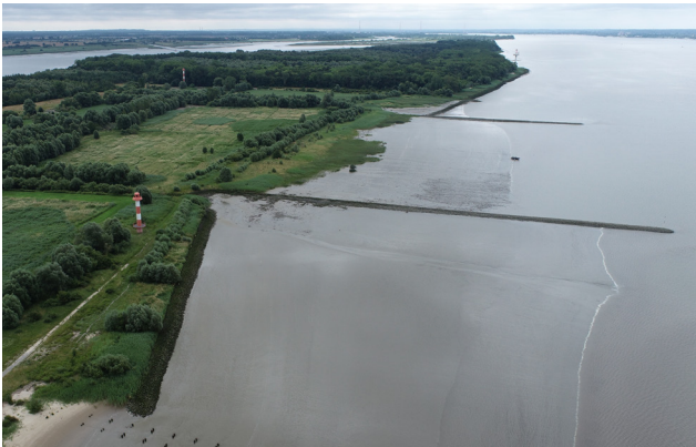
Figure 8: Revetments and groyne system for embankment and foreshore stabilisation against ship waves at Pagensand in the Lower Elbe Estuary. Central groyne field without revetment. Source: Federal Waterways Engineering and Research Institute (BAW).
