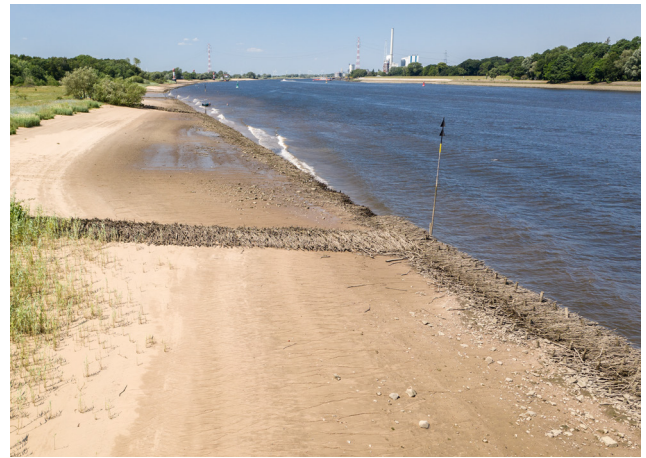
Figure 11: Brushwood berm and groyne are successfully employed to retain the beach and vegetation belt at Warflether Sand in the Lower Weser Estuary, Germany. Source: Federal Waterways Engineering and Research Institute (BAW).
