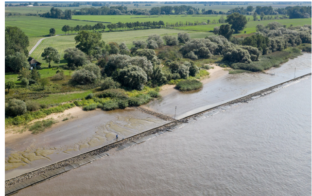
Figure 9: Nearshore composite berm for load reduction in combination with brushwood groynes for sediment retention at Harriersand in the Lower Weser Estuary, Germany. Source: Federal Waterways Engineering and Research Institute (BAW).
