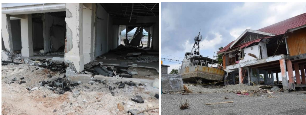
Figure 2: Concrete debris impacts (left) and vessel impacts (right) (photos taken by Jacob Stolle).
