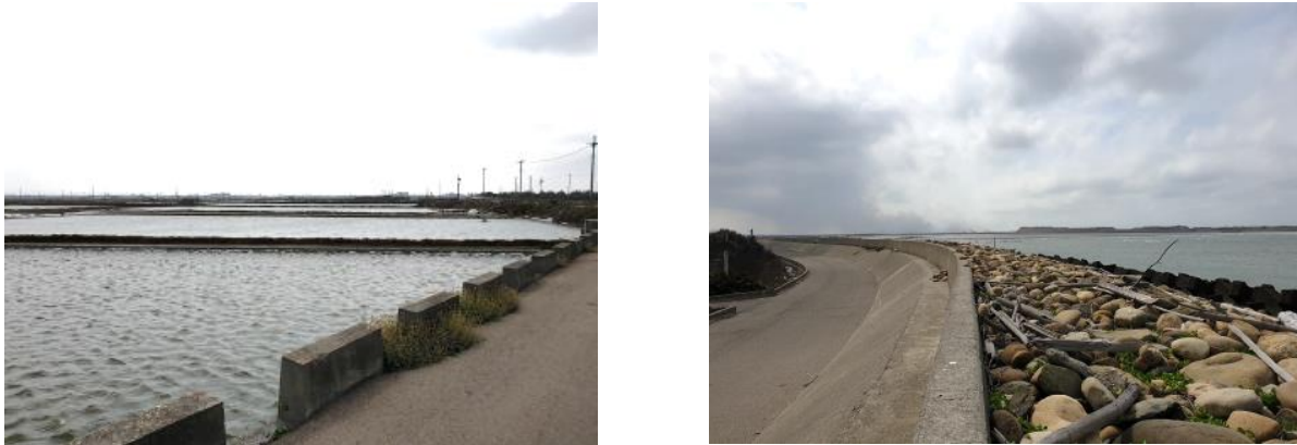
Figure 2: Left. Fish farms in Yunlin. Right. Coastal protection structures in Yunlin
