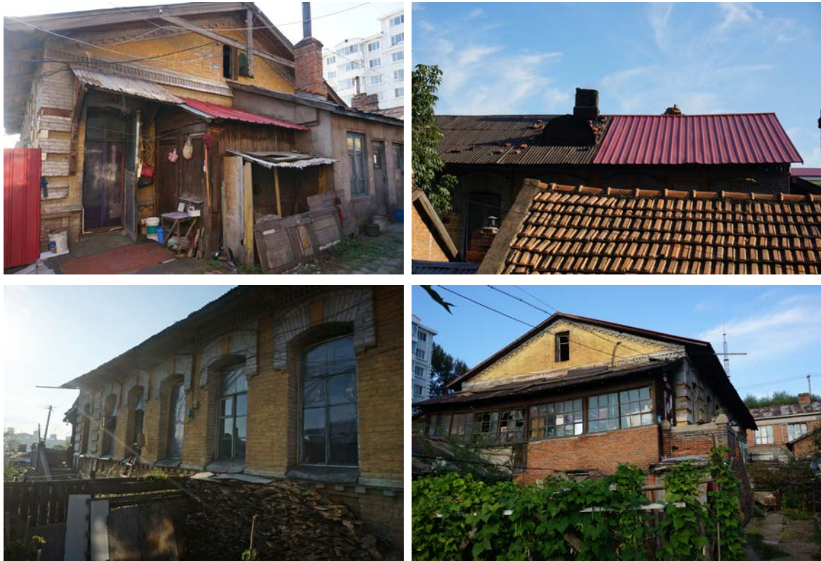
Figure 7 Environment of historic buildings
