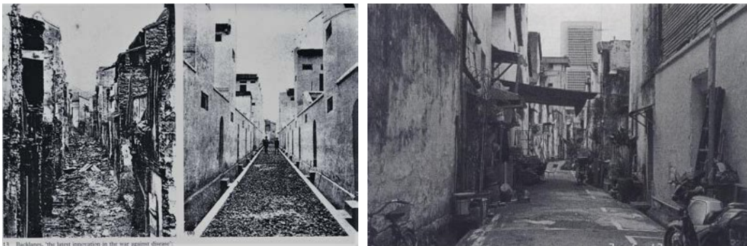
Figure 5 (Left): Yeoh, Brenda S. A. 'The latest spatial innovation in the war against disease' according to the government, the photo shows the demolition of the back of the shophouses to create back-lane. [Singapore: s.n, 2003]
