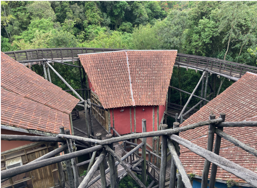
Fig. 4. The Free University of the Environment was built with traditional construction methods
