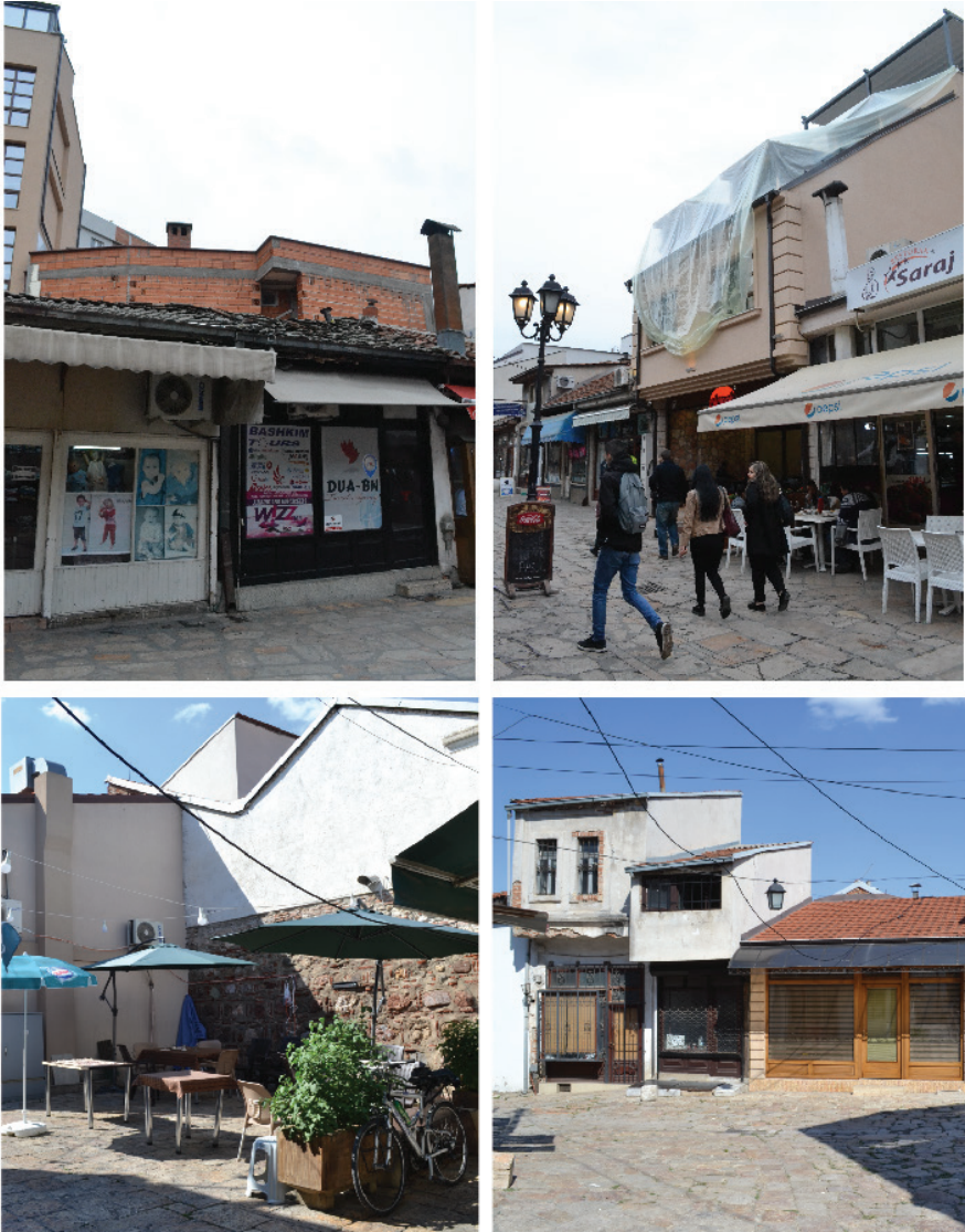
Fig. 1. Strict regulations vs. loose control leads to informal and illegal appropriations
