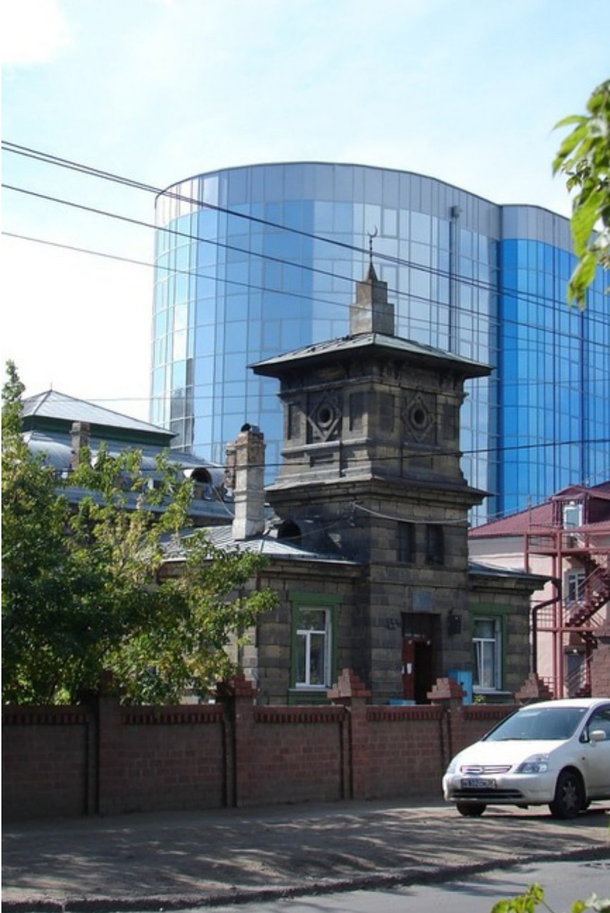
Fig. 2. Irkutsk: mosque in the Karl-Liebnecht Street in front of a new glass facade which disturbs the perception of the historical monument
