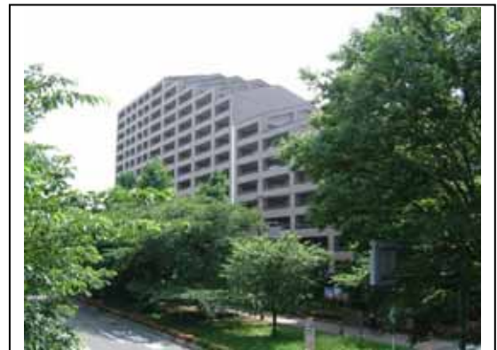
Photo 1. An eighteen-storey apartment along Daigaku Street
