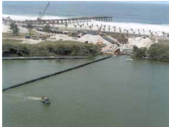
Illustration 9. Sanitary works in Lagoon Marapendi. Source: CEDAE, 2006.
