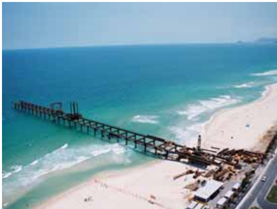
Illustration 8. Construction of submarine emissary. Source: CEDAE, 2006.
