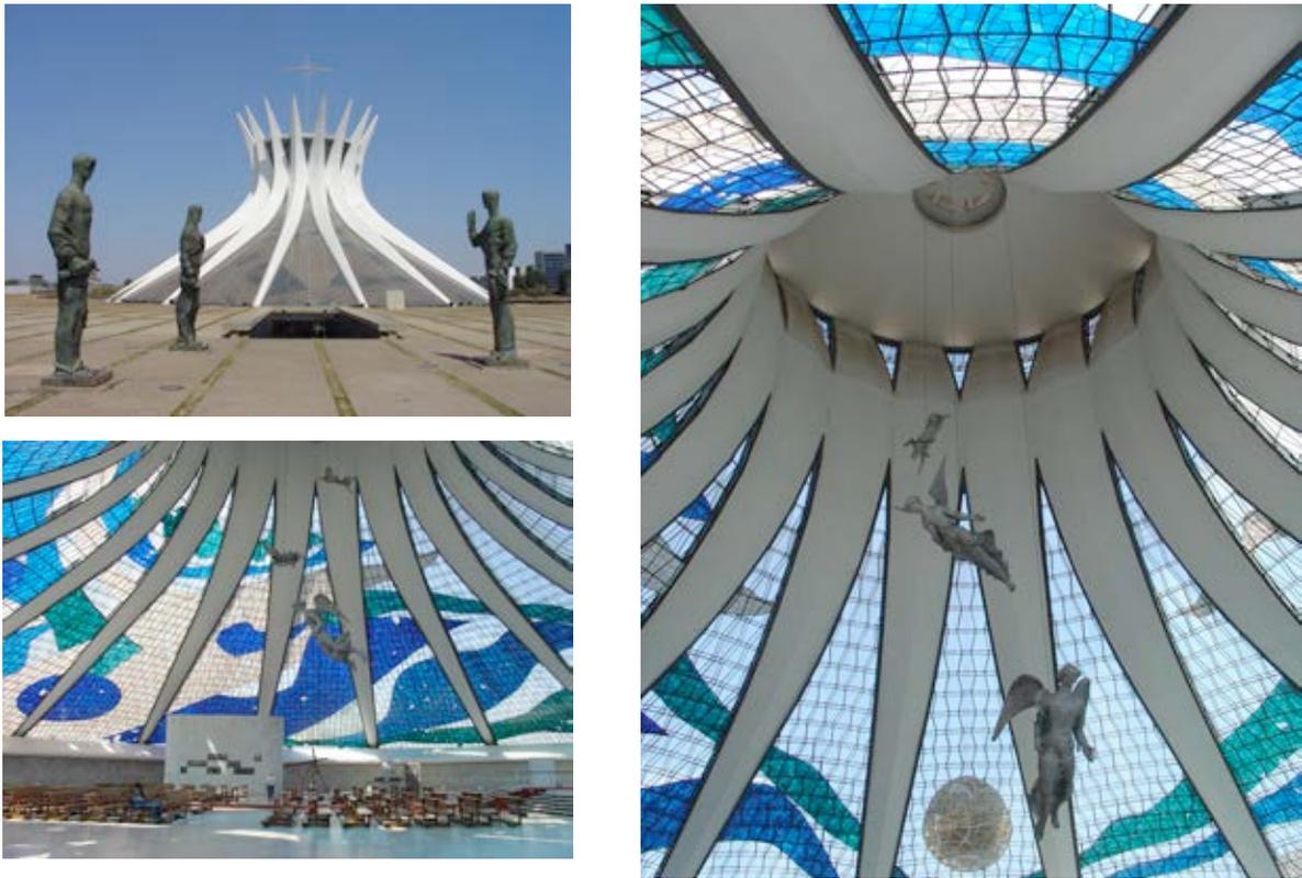
Figures 5, 6 and 7: Brasilia Cathedral, present state. View towards the outer access ramp, interior devotional space bathed in daylight, and detail of the compression ring, roof slab and glazed curtain walls among the piers
