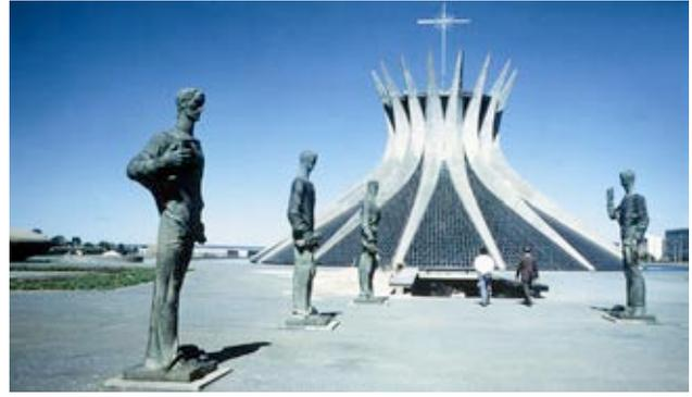
Figure 3: Brasilia Cathedral, with exposed concrete structure and lateral sheathing between the piers
