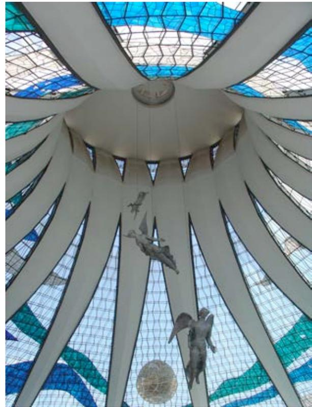
Figures 5, 6 and 7: Brasilia Cathedral, present state. View towards the outer access ramp, interior devotional space bathed in daylight, and detail of the compression ring, roof slab and glazed curtain walls among the piers
