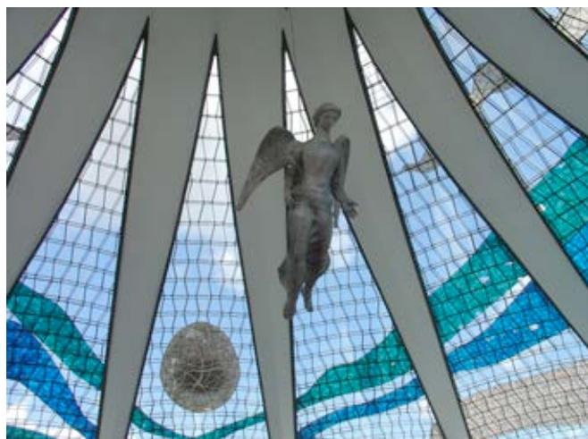
Figure 11: The spatial frame between the piers allows the fastening of two layers of glazing on the upper and lower hexagonal webs of the truss (my photo).
