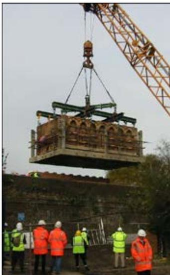
Figure 5. A section of the Waterpoint being lowered into its new position, November 2001
