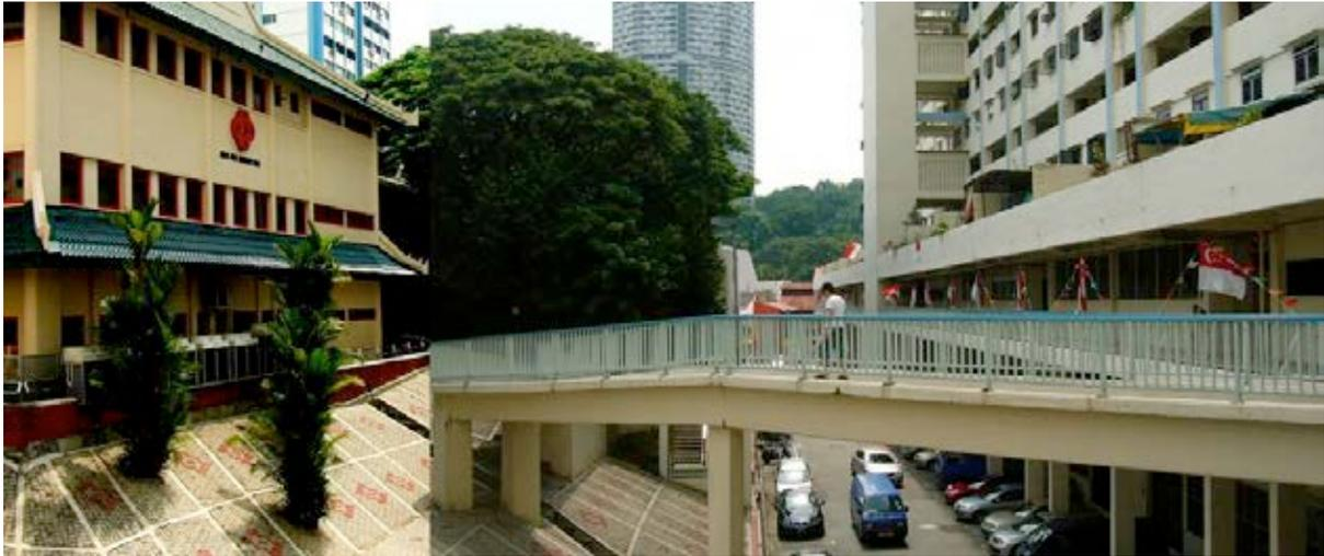
**Fig.17** High-level linkages that bridge the surrounding housing blocks to the central communal area
