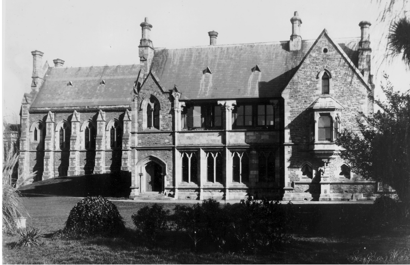
Figure 5 Canterbury Provincial Council Buildings showing the Council Chamber (left) and Refreshment Rooms added in 1864-65. (Photo: Alexander Turnbull Library, Wellington)
