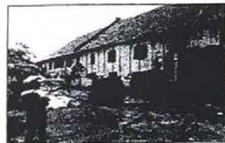
Condition of A and B Buildings
