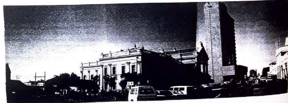
FIG 2 Kimberley Market Sq with Town Hall and new PO tower.
