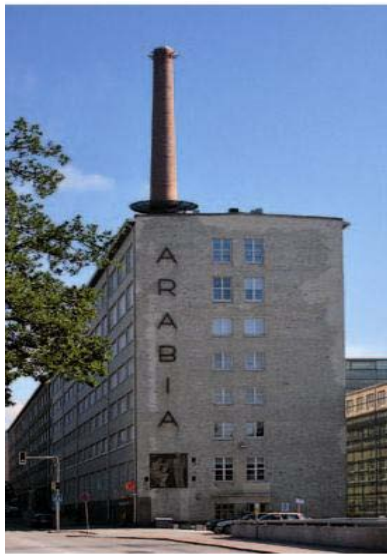
Figure 6. The Arabian old factory chimney(from: http://www.arabianranta.fi )
