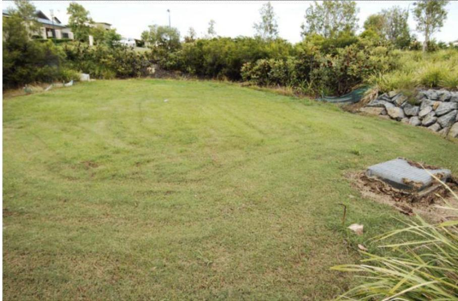
*Figure 1 Typical stormwater detention basin*
