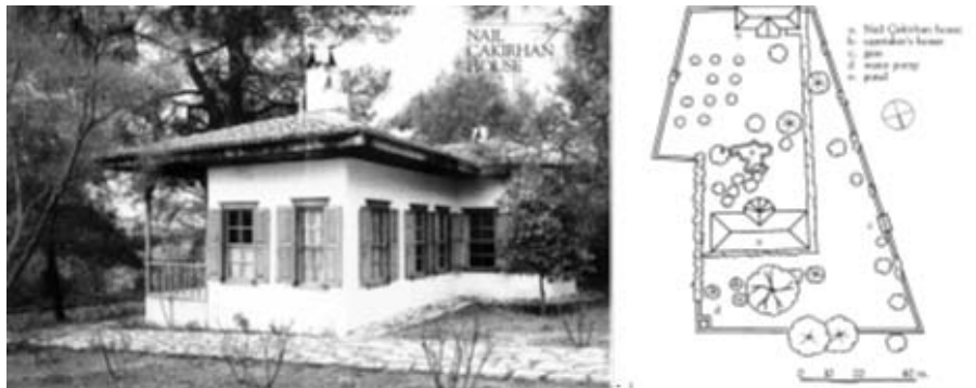
Figure 2 Çakırhan House (Cantacuzino, 1985) the location of the care taker house is against the legislations. There should be a minimum distance between the block and the border of the lot
