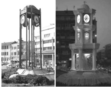
Figure 4. Heykel Clock Tower, before and after reconstruction
