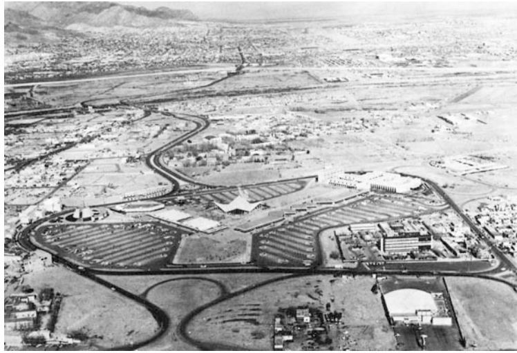
Figure 5. Aerial imagen of ProNaF's Commercial Center in construction in the 1960s. Anonymous author.
