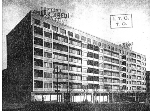
Figure 5. Istanbul Municipality - Emlak Kredi Bank Apartment Building on Atatürk Boulevard, Istanbul Municipality Housing office, 1954-1957.
