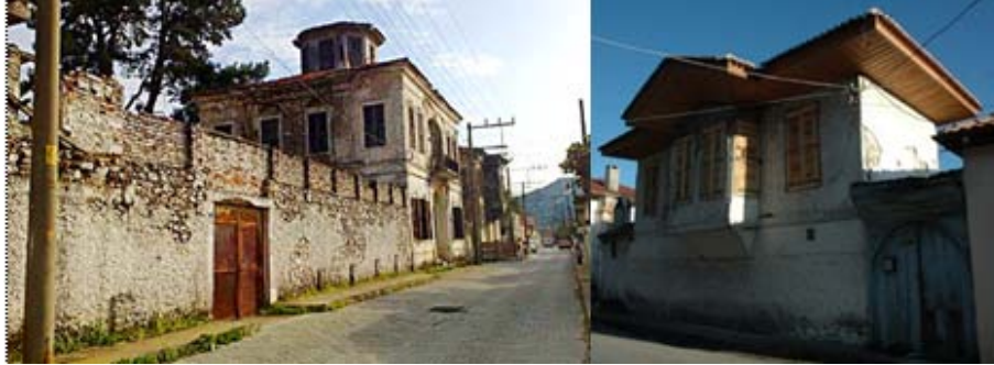
Figure 3 Traditional Ula House (Photo: Left Muğla Kültür Turizm İl Müd. Right Ula Municipality)
