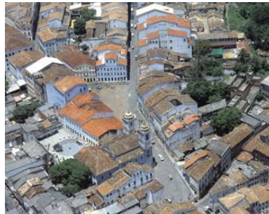
Figure 10: aerial view of Pelourinho
