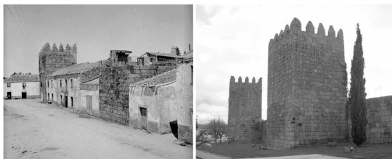
Figure 7 - City walls of Trancoso, before and after the interventions (source: IHRU).
