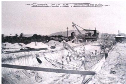
Figure 02 - Channel 4 under construction. Source: SÃO PAULO, 1925.
