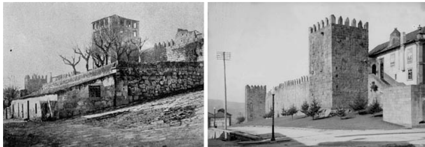
Figure 3 - City walls of Oporto, before and after the interventions (source: IHRU).
