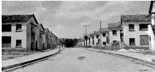
Figure 3 A view from the main street and the two-story high independent units row in 1952
