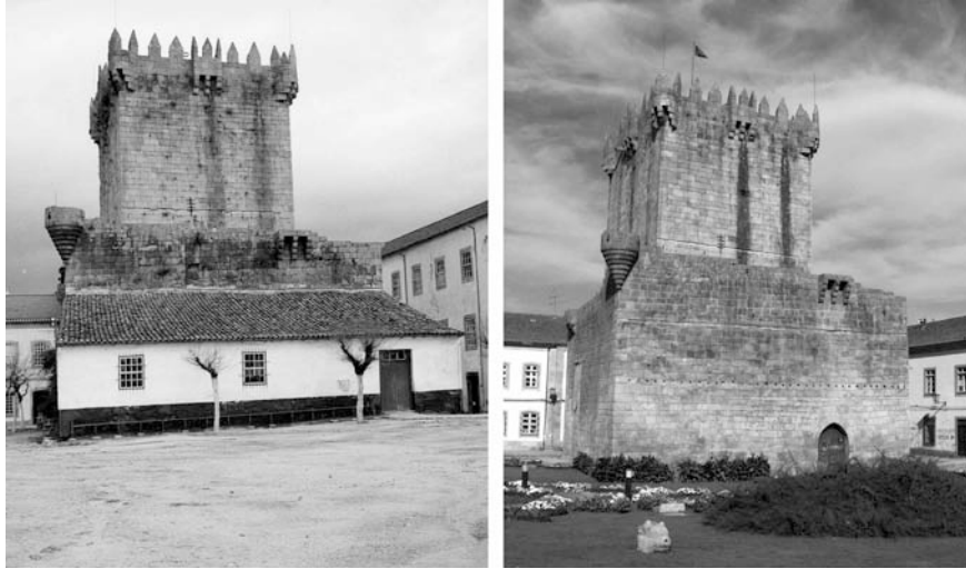
Figure 8 - Castle of Chaves, before and after the interventions (source: IHRU).
