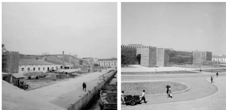
Figure 6 - City walls of Lagos, before and after the interventions (source: IHRU).
