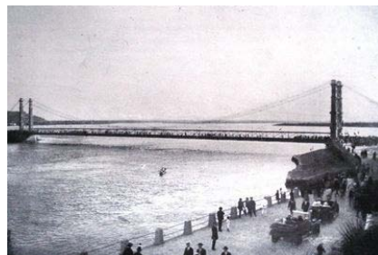
Figure 05 - Inauguration of the Suspension Bridge on May 21, 1914. Source: SÃO PAULO, 1916.
