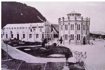
Figure 04 - Santos Sanitation - Terminal Plant and Prevention Plant. Source: SÃO PAULO, 1912.
