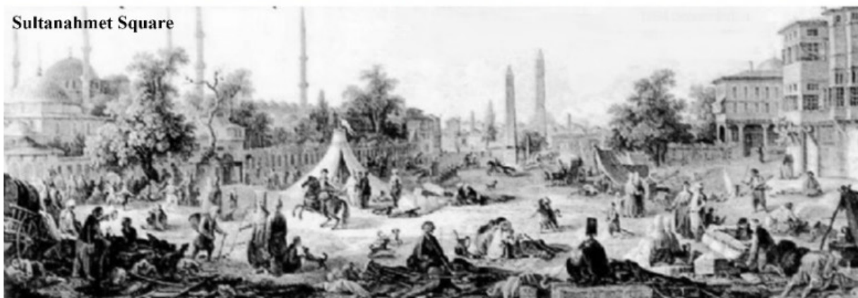
FIGURE 2 The earthquake of 1894. Damaged Historic Neighborhoods and Monumental Structures
