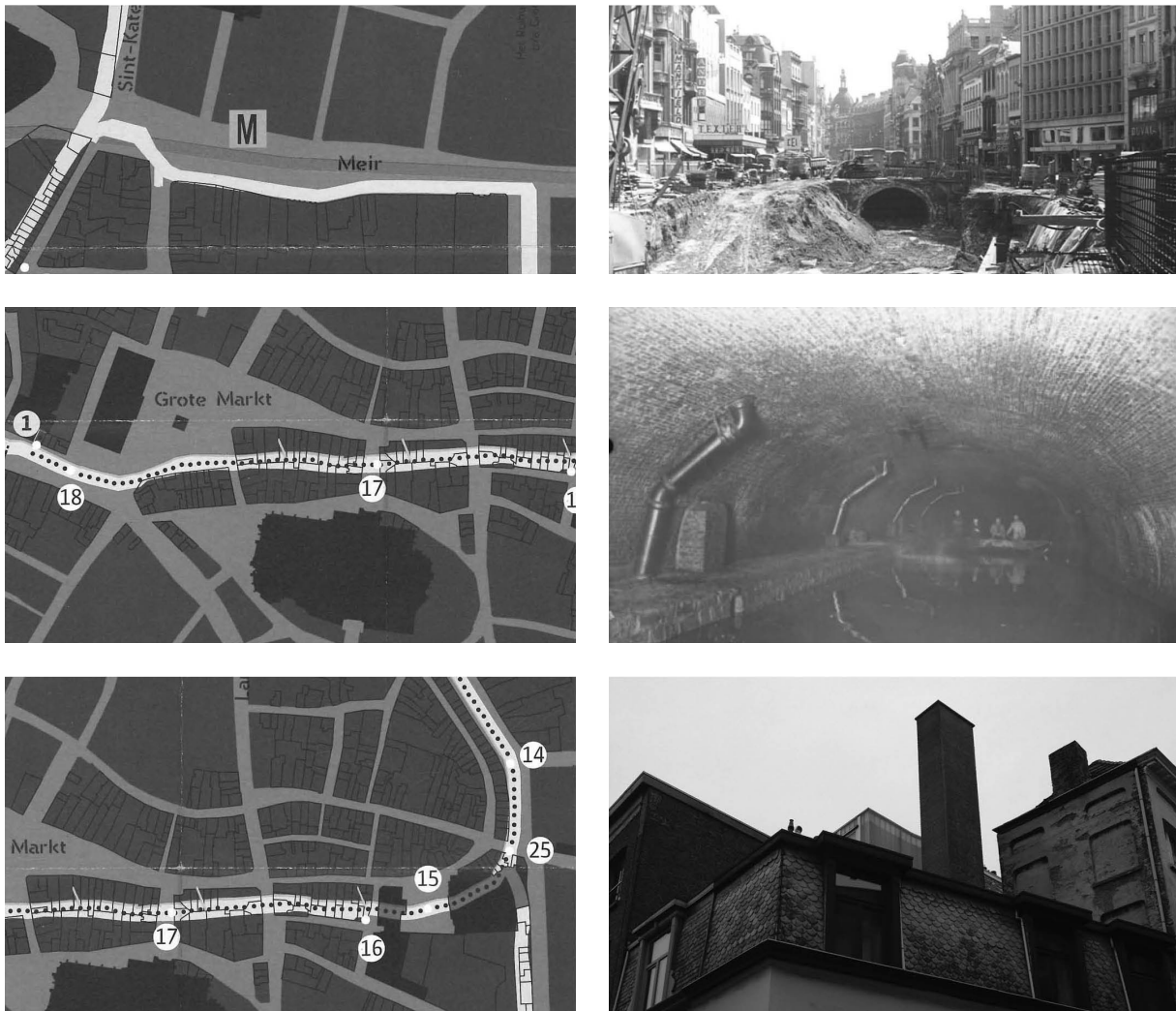
FIGURE 4 The Ruien tunnels were partially recovered and rerouted for the construction of the premetro in 1970 (top). For a large part, houses were built on the covered Ruien. Their sewage was directly connected to the underground Ruien network (middle). Where the Ruien were transformed into streets, such as the Minderbroedersrui, the width of the street is quite generous, based on its subterranean ‘water size’ (bottom left). Above ground, elements such as ventilation shafts offer clues of the now entirely covered Ruien network (bottom right).
