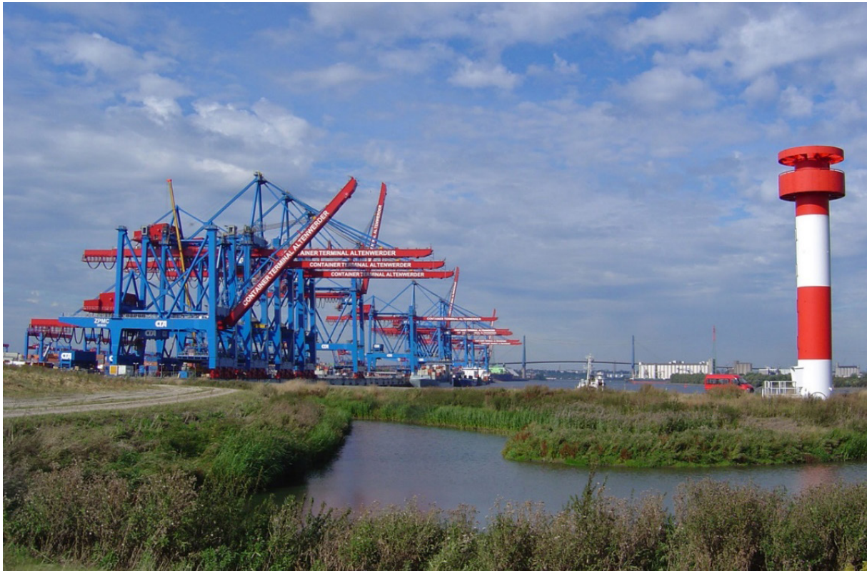
FIGURE 5 Container terminal Altenwerder in 2004
