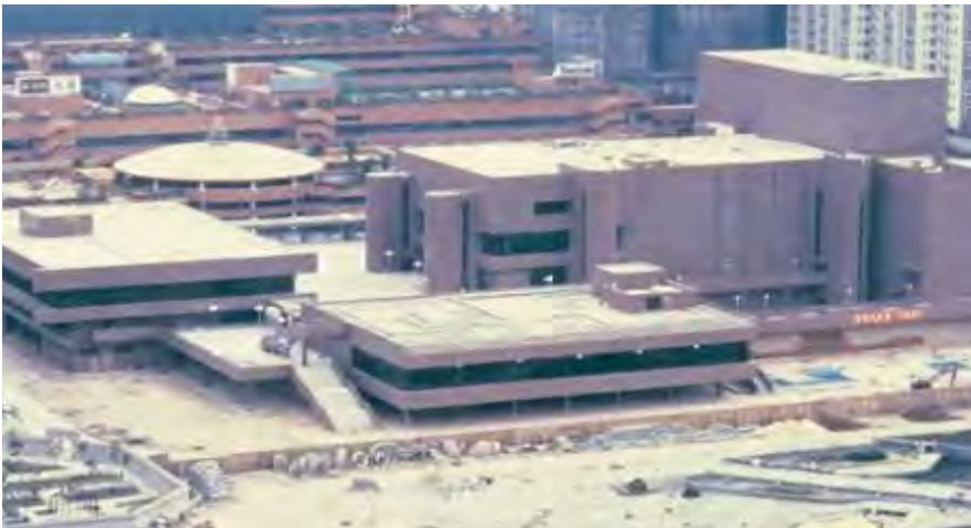
Fig. 5. Shatin Town Hall in construction (1986)
