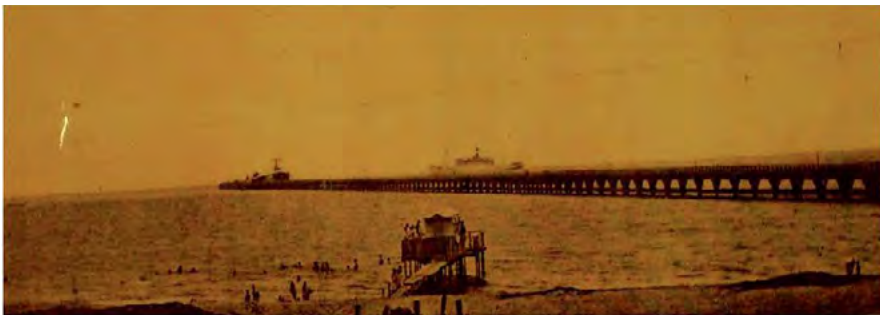
Fig. 2. Archive of the Romantic Museum of Barranquilla. Puerto Colombia Dock, after the concrete casing works have been completed. 1894.
