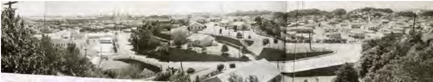
Fig. 8. Old photo of the District 2 on Wadayama hill (planned area of the hilltop park)
