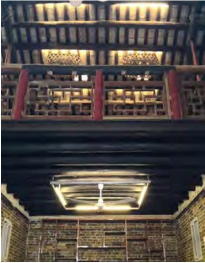
Fig. 5. Example of using recycling materials for interior renovation for a traditional house. (Photo by author, 2015)
