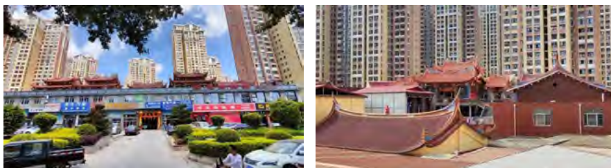
Fig. 1. Temples on the rooftops. Putian, Fujian province, China. Three temples of villages were built on the rooftop of the bungalow together, the function in the bungalow is commerce.
