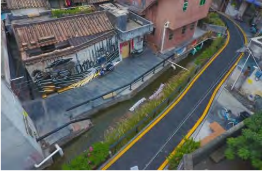
Fig. 8. Post-renovation assessment of road conditions.
