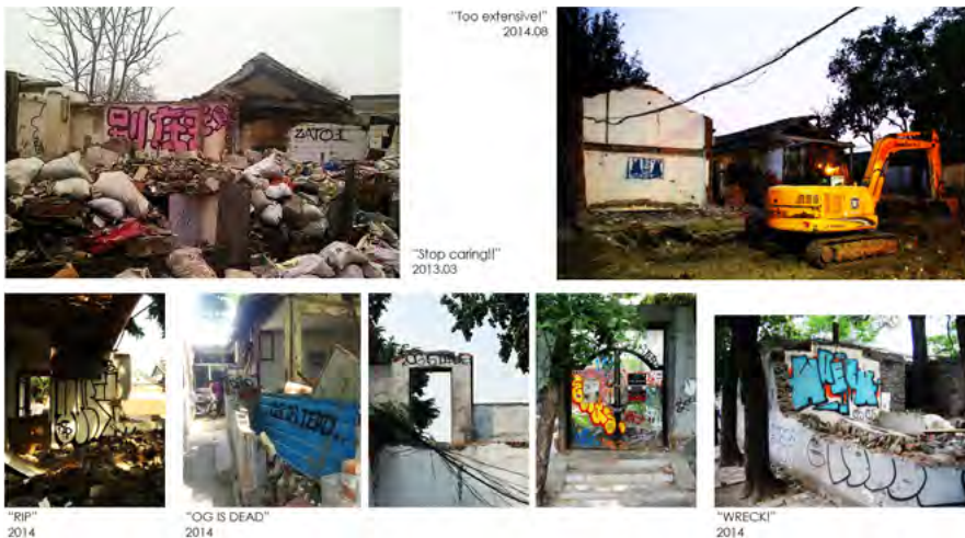
Fig. 6. Series of graffiti appearing on the BDT demolition site from 2013-2014.
