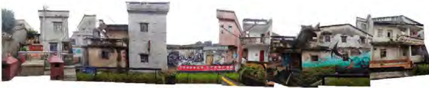
Fig. 7. Façade of border buildings along the Longjin River after renovation. The walls are adorned with frescoes crafted by artists.
