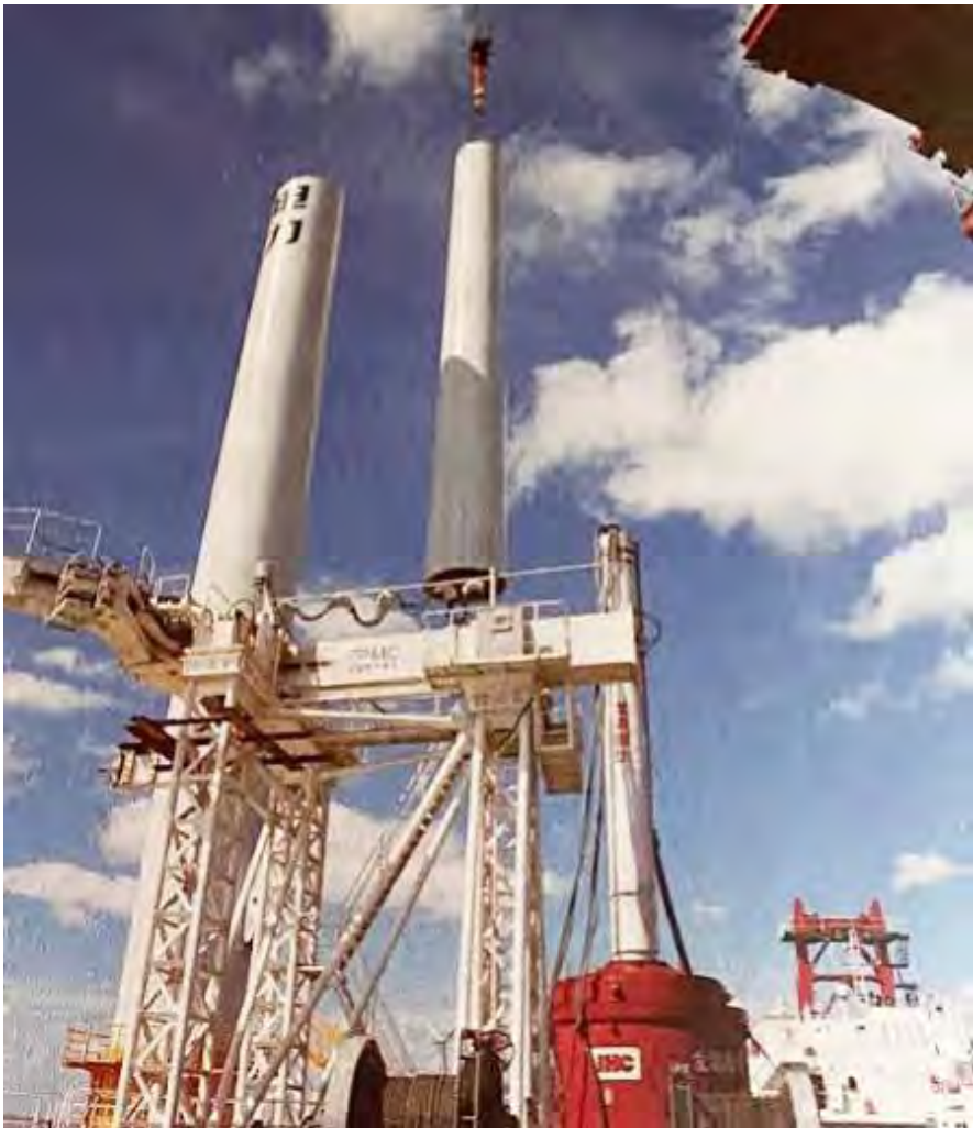
Fig. 5. Construction of the Rudong offshore wind farm.
