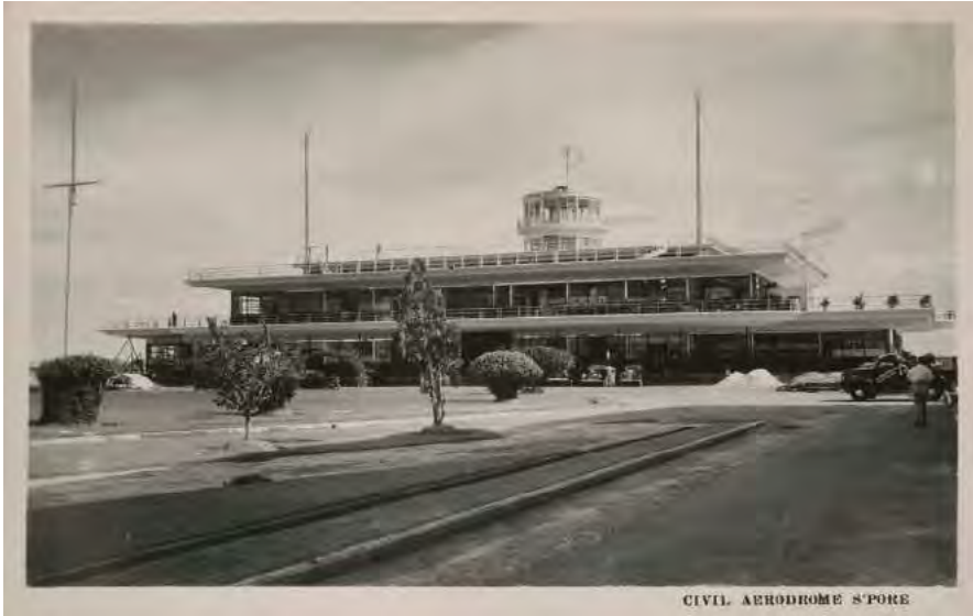
Fig. 2. View of Kallang Airport Terminal Building from ceremonial tear shaped drop off, 1940s 7
