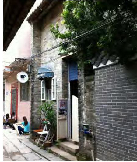
Fig. 6. Example of new program for a traditional house. (Photo by author, 2015)
