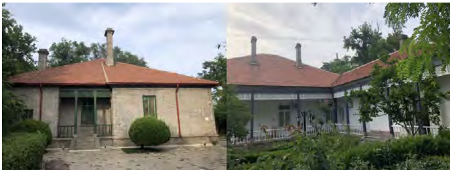
Fig. 6 & 7. Former British Consulate; Former East Customs Tax Department
