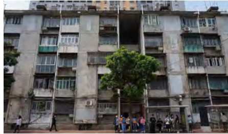
Fig. 8. Resettlement Housing of Ilha Verde Area. Back Façade. © Niccolò A. Galliano, 2023.
