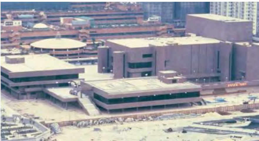
Fig. 5. Shatin Town Hall in construction (1986)
