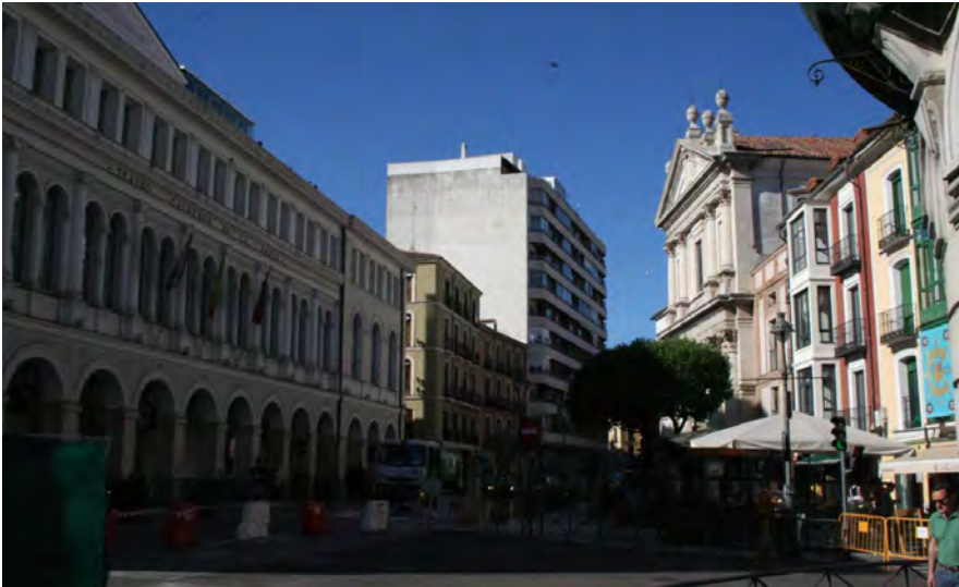
Fig. 6. Photos of calle Angustias showing the alignment reform at two different times, in which the rupture of the new building at n° 7 and 9 is visible.
