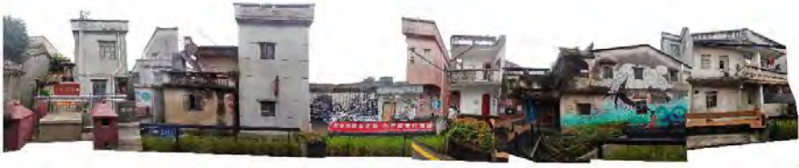
Fig. 7. Façade of border buildings along the Longjin River after renovation. The walls are adorned with frescoes crafted by artists.
