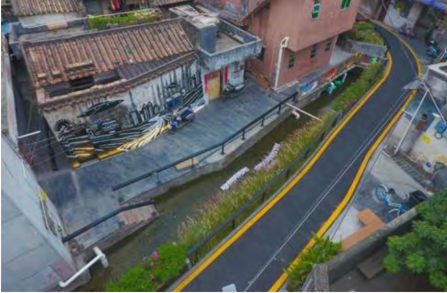
Fig. 8. Post-renovation assessment of road conditions.
