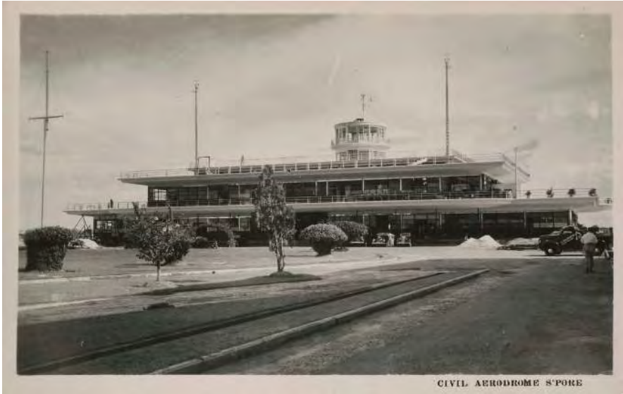
Fig. 2. View of Kallang Airport Terminal Building from ceremonial tear shaped drop off, 1940s 7
