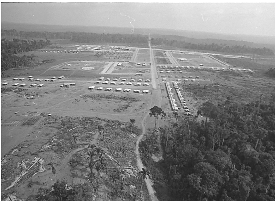
Fig. 2. Aerial view of one of the Transamazonian new towns, 1970s.
