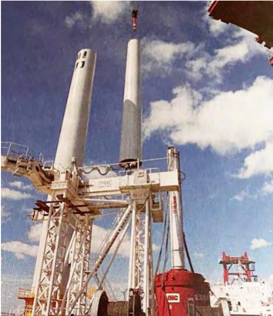
Fig. 5. Construction of the Rudong offshore wind farm.
