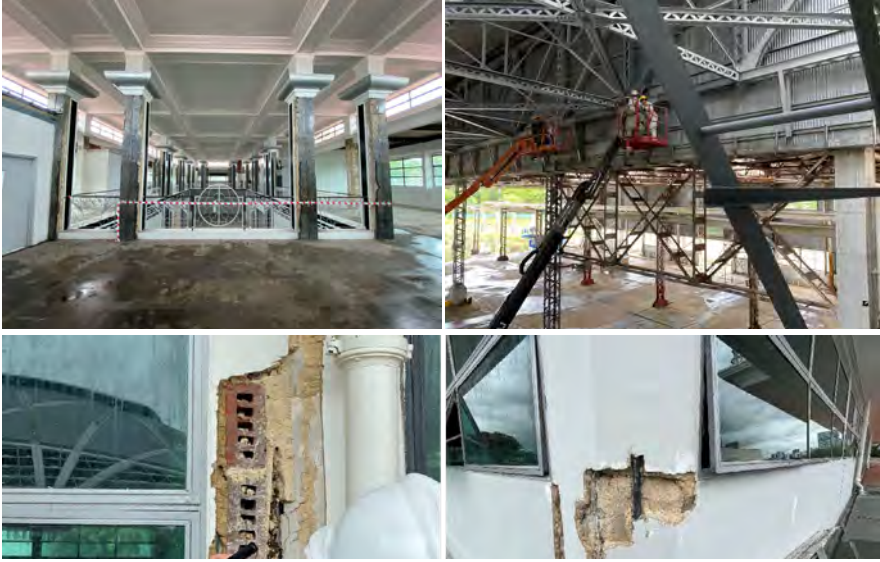
Fig. 13. Clockwise (L to R) - Level 2 of Terminal Building with exposed columns, Workers in the midst of repainting steel trusses of Hangar A, External wall of Terminal Building stripped of plaster exposing brickwork, External wall of Terminal Building stripped of plaster exposing block masonry, reinforced concrete structure and embedded piping. (Source: DPA)
