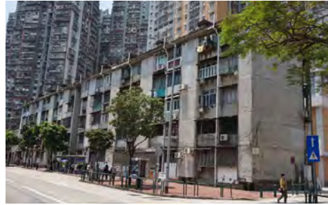
Fig. 2. Resettlement Housing of Ilha Verde Area. Back Façade. © Niccolò A. Galliano, 2023.
