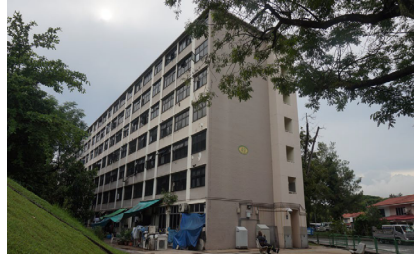
Fig. 18. Queenstown New Town 45-48-49 Housing Blocks. © Niccolò A. Galliano, 2023.
