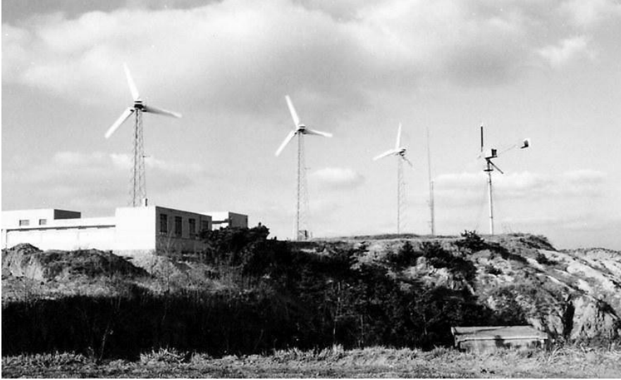
Fig. 3. Wind turbines in Rongcheng, Shandong.
