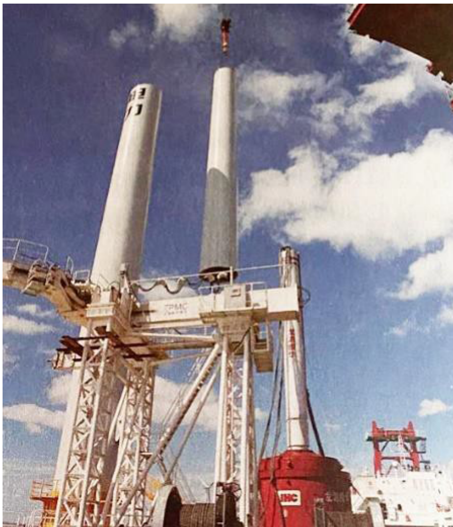
Fig. 5. Construction of the Rudong offshore wind farm.
