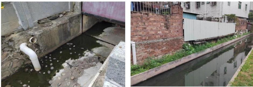
Fig. 13 & 14. Comparison between the renovated and unrenovated runoff
