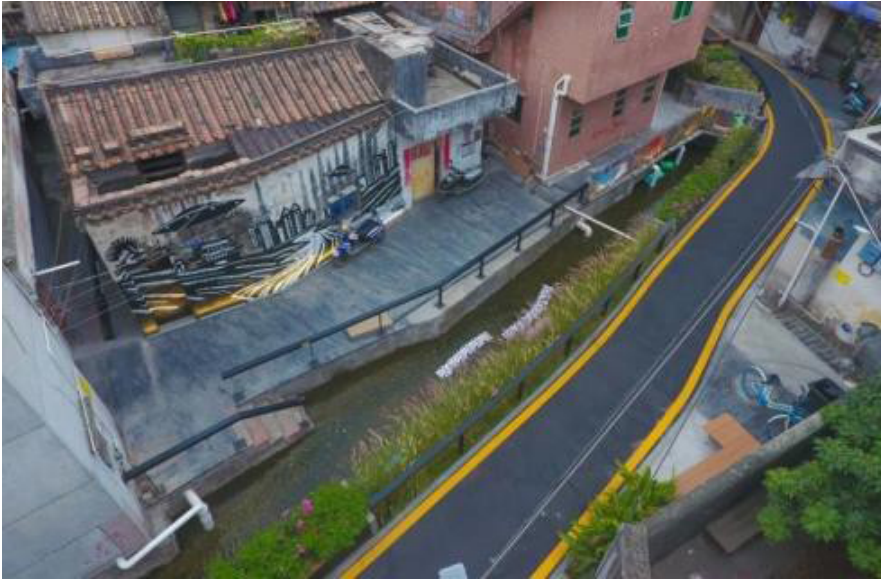
Fig. 8. Post-renovation assessment of road conditions.
