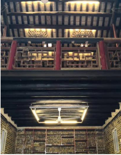
Fig. 5. Example of using recycling materials for interior renovation for a traditional house. (Photo by author, 2015)
