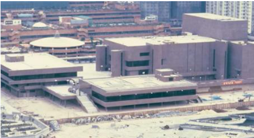
Fig. 5. Shatin Town Hall in construction (1986)
