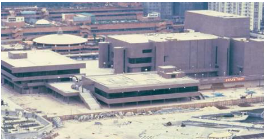
Fig. 5. Shatin Town Hall in construction (1986)
