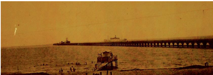
Fig. 2. Archive of the Romantic Museum of Barranquilla. Puerto Colombia Dock, after the concrete casing works have been completed. 1894.
