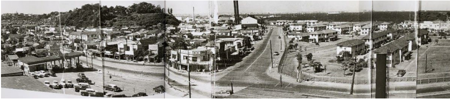
Fig. 7. Old photo of the District 1 on the right and Japanese houses on the left
