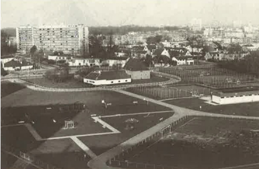
Fig. 1. Apartment building of Etrimo in the southern border of Antwerp, ca. 1980. 3
