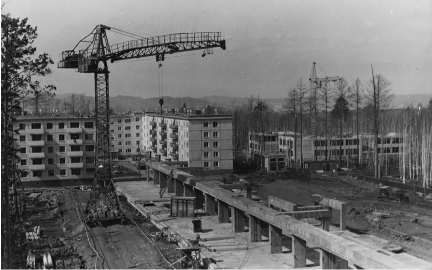
Fig. 1. Towards the Socialist City: Construction of the 3rd Micro-district in Ust-Ilimsk 1978.
