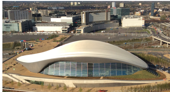
Figure 2 London Aquatic Centre designed by Zaha Hadid Architects
