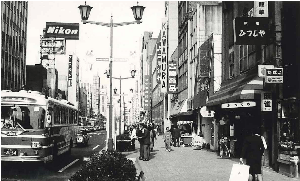
Figure 9: Ginza Street after large-scale construction (1968) Source: Ginza Street Association
