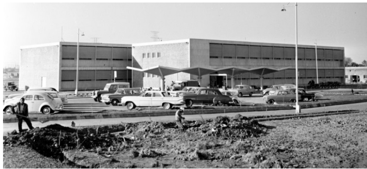
Figure 8: National Company of South oil fields in Ahwaz Source: Iranian Oil Museum Archives
