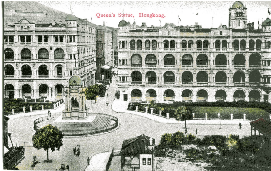
Figure 3: Statue Square, probably during the first decade of the 20th century when construction was still going on around its peripheries (postcard published by M. Sternberg of Hong Kong, author's collection). The formal arrangement of the square, with the greenspaces cordoned off from public access by railings, was more a place for celebration of empire than leisurely occupation.
