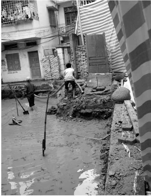
FIGURE 6 Septic tank emptying
