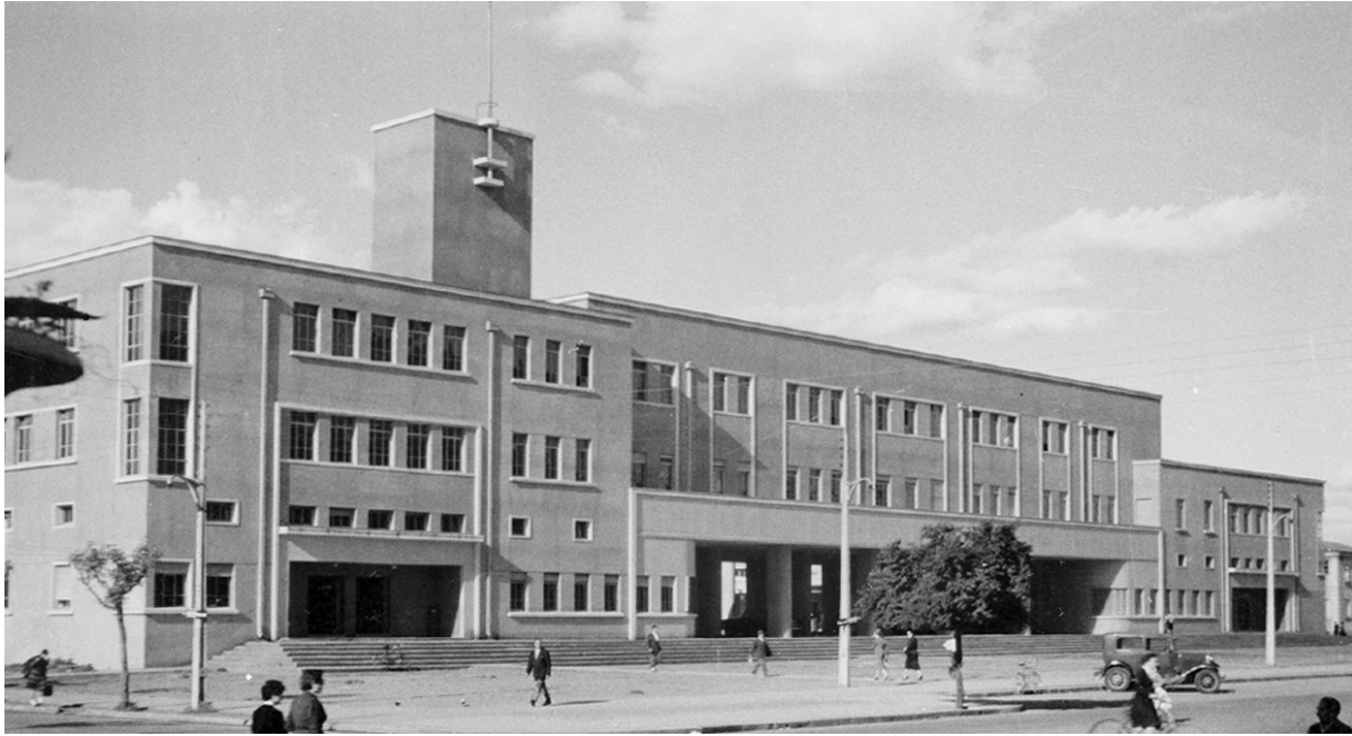
FIGURE 6 Public Services and Administration building, by Benavente and Morales (1940), the main building of Chillán new civic centre.
