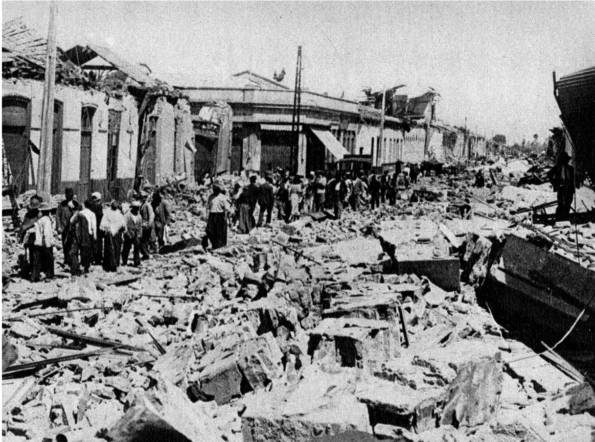
FIGURE 1 Chillán, 1939: “A painful procession”. People walking in a street piled with waste materials from destroyed buildings, the morning after the earthquake.
