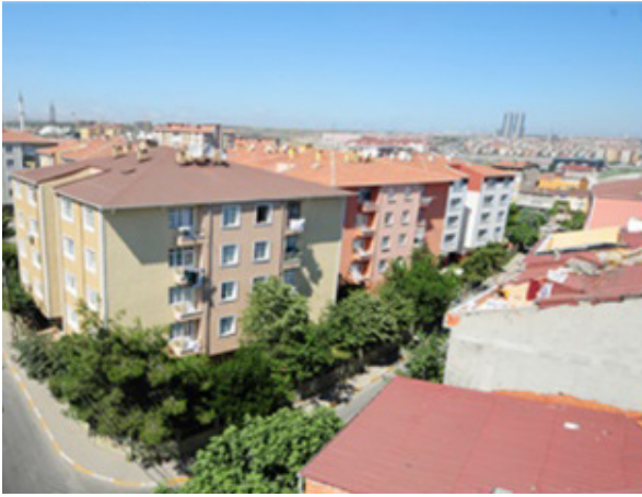
1 Barinkent Housing Estate: Apartment blocks before
