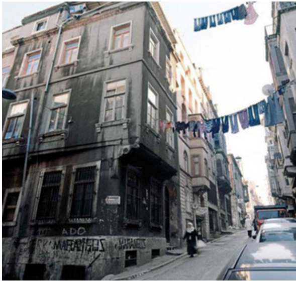
1 Historic pre-20th century neighbourhoods- now occupied by the urban poor; high earthquake risk locations, which are increasingly vulnerable to gentrification.
