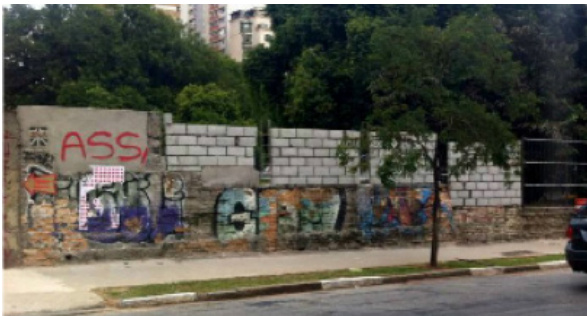
After Setin and Cyrela: All gates are sealed
