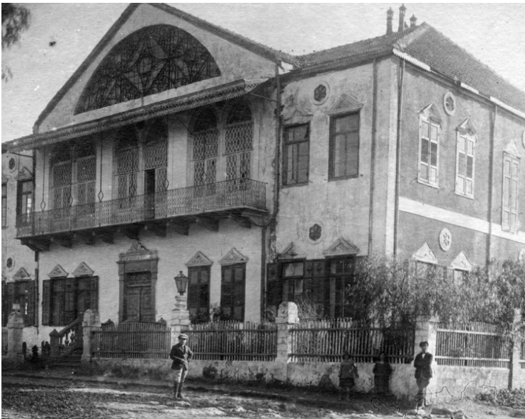
FIGURE 3 Zichron Ya'akov, Administration House,
