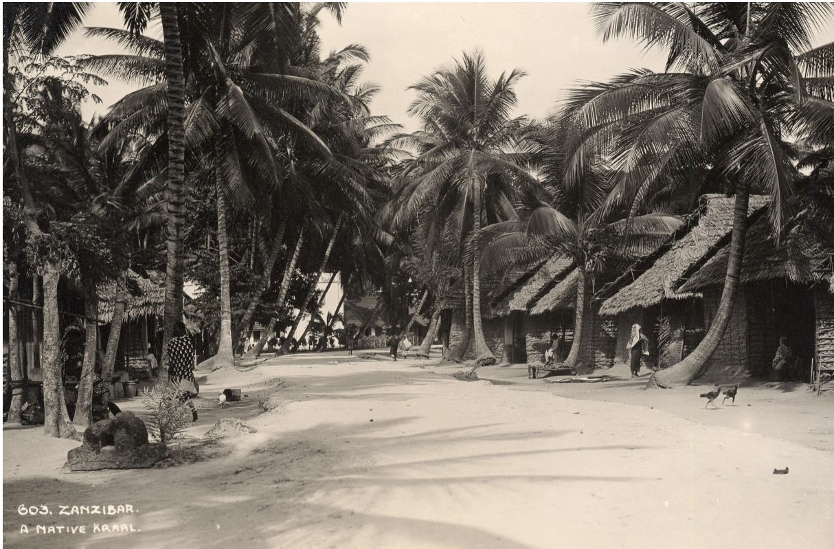
FIGURE 4 A typical street in Ng'ambo, around 1900. Single storied Swahili houses with makuti roofs and a double storied flat roofed building in the background.
